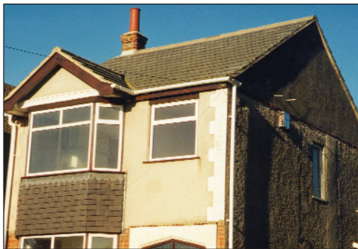
Closer view of main windows
